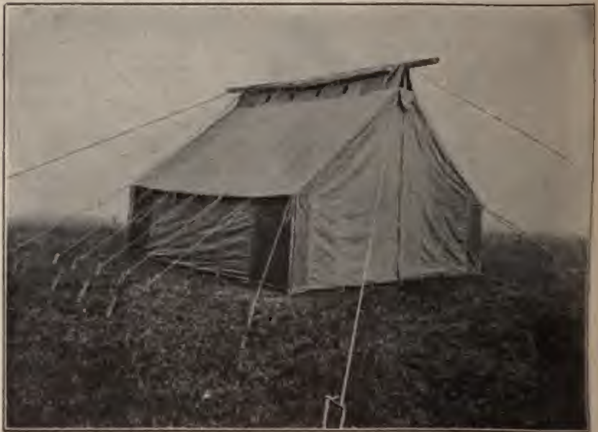
FIG. 196.—Hospital tent, tropical, showing ventilation of attic.
